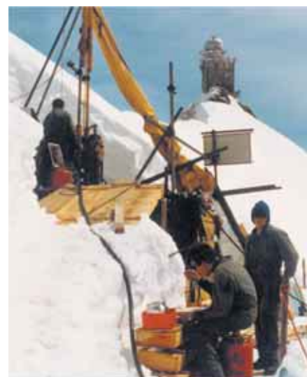
Pendelbohrung/Staumauer Grande Dixence ▶
